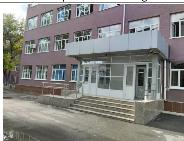
Ramp in Building 5
