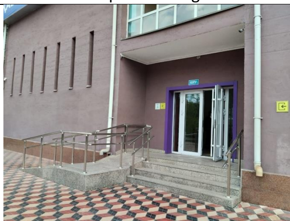
Ramp in Building 3
