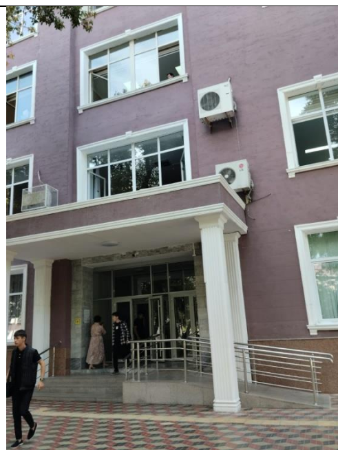
Ramp in Main Building
