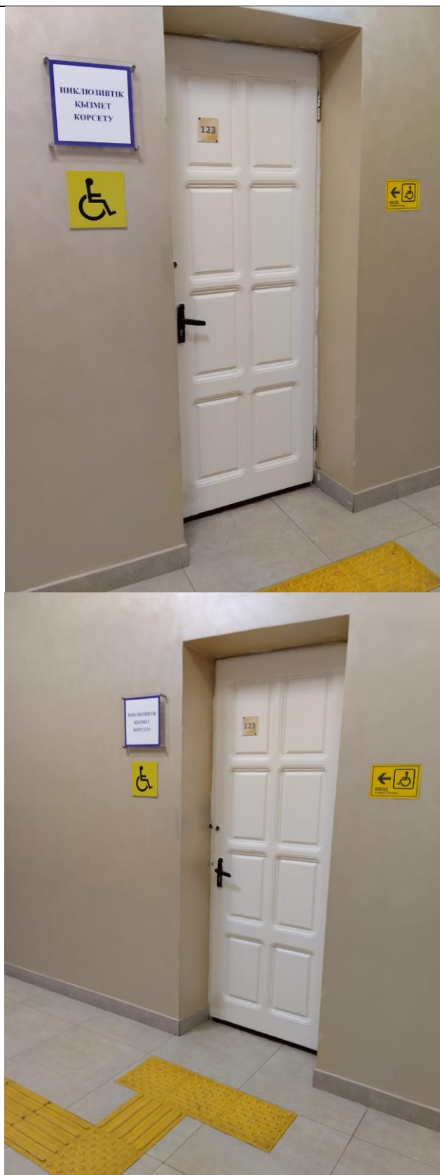
Auezov University office “Inclusive service delivery” with tactile tiles on the floor and vertical signs on the wall
