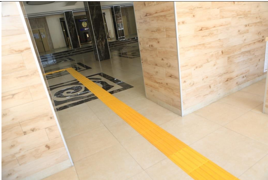
Tactile floor tiles for the visually impaired and disabled. Available in every building
