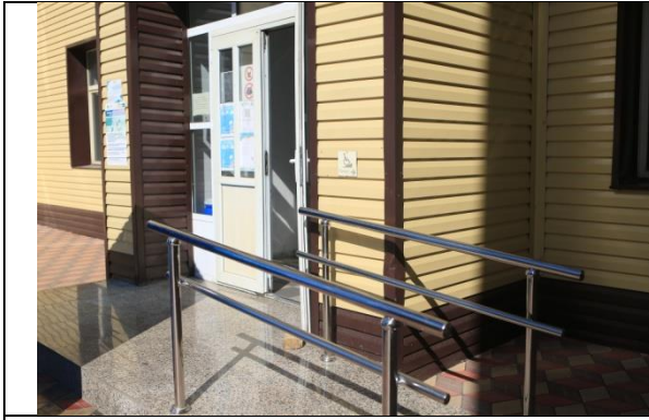
Ramp in Building 4
