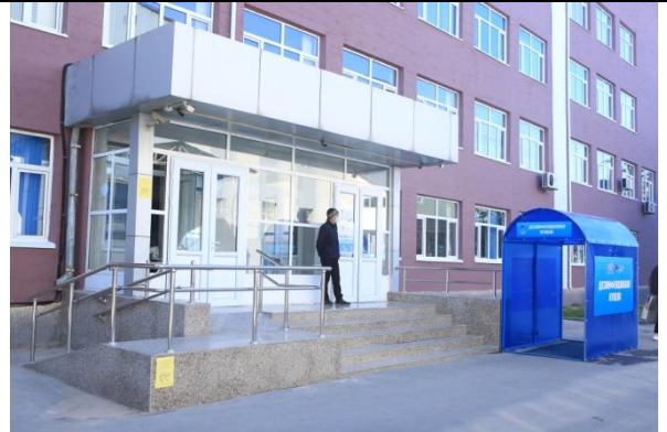
Ramp in Building 5
