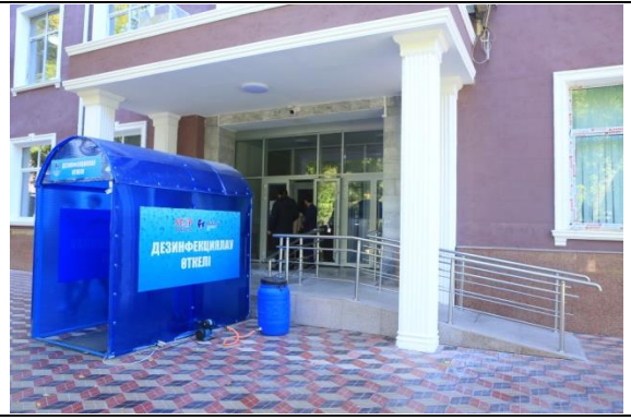
Ramp in Main Building
