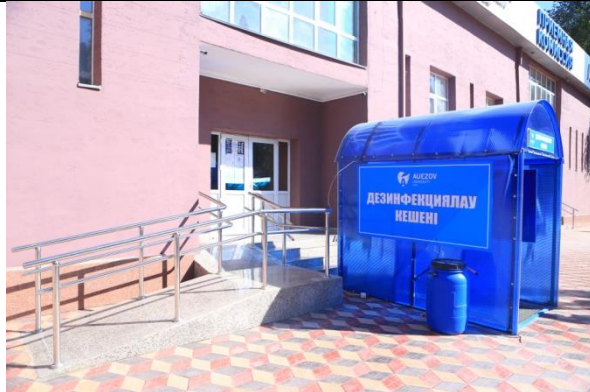
Ramp in Building 3
