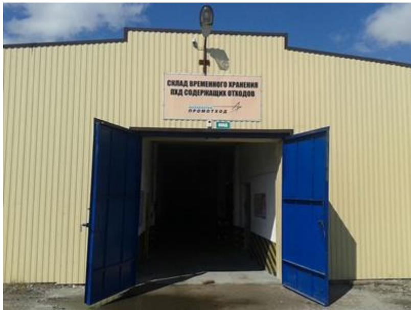
Warehouse for temporary storage of hazardous waste of the Company "Promothod Kazakhstan"
