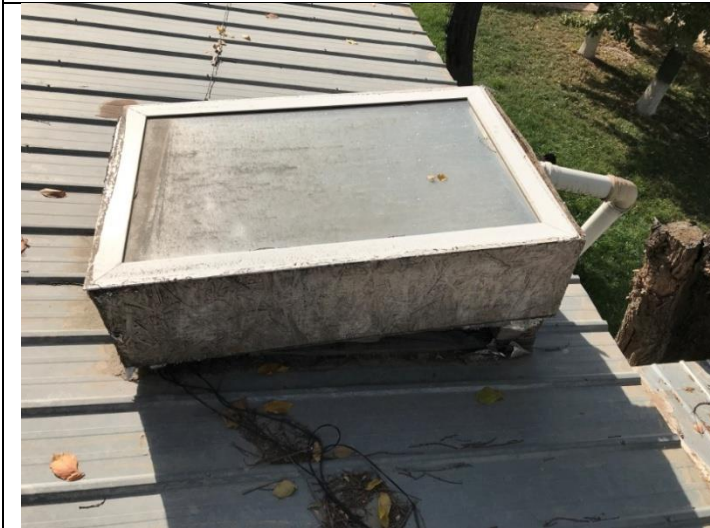
Campus 1. Heliocamera for solar energy accumulation
