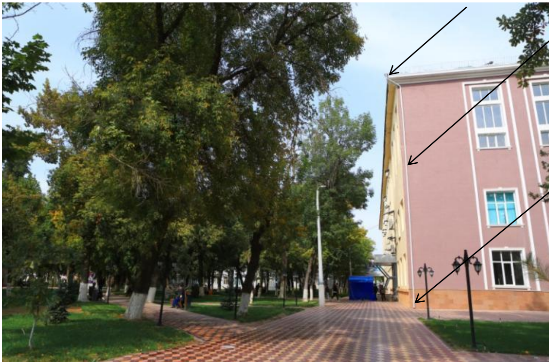
Showery runoff from the roof of the main campus building 1
