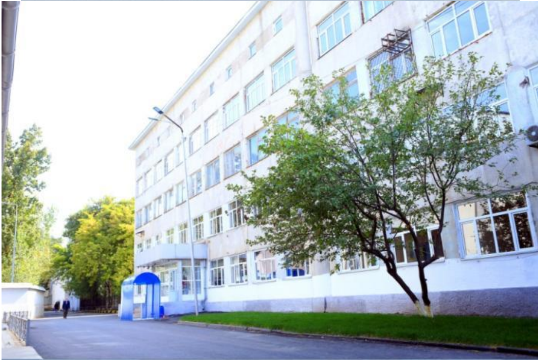
Natural lighting thanks to the large number of panoramic windows.
