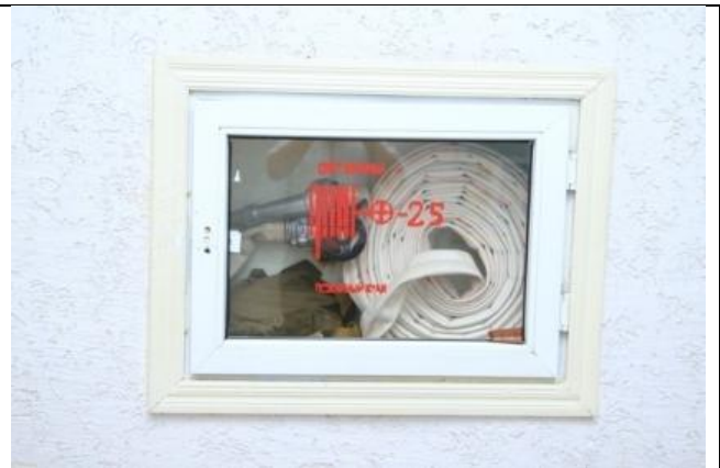
Fire hydrant inside the building
