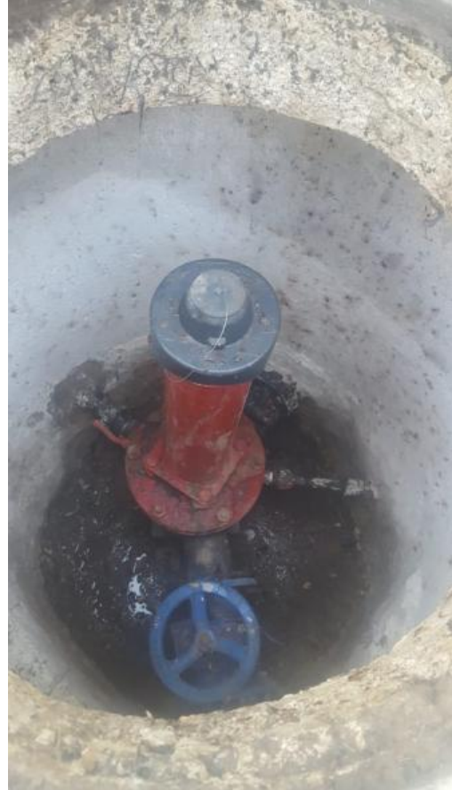
Fire hydrant inside the building
