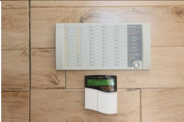
Alarm control panel in the main building
