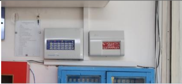
Alarm control panel in the main building
