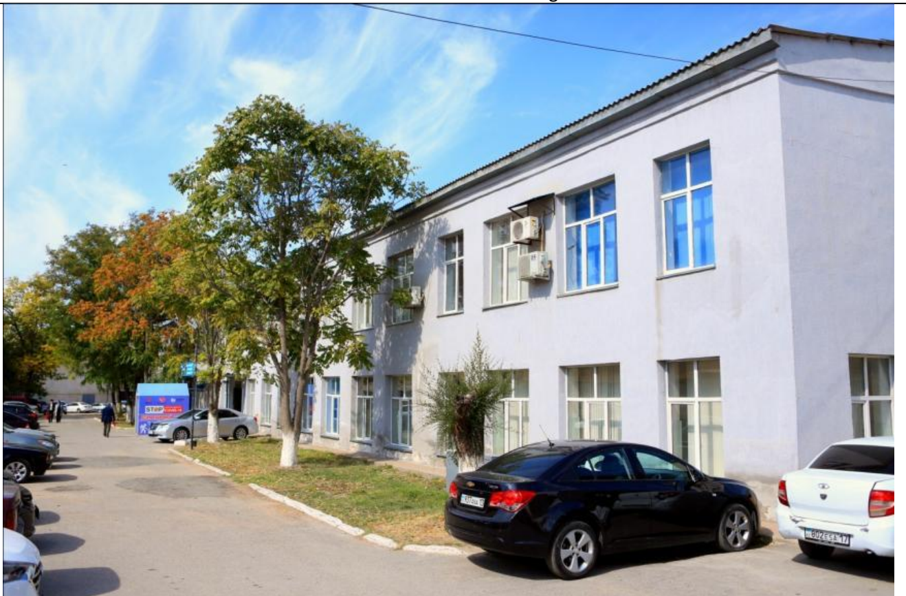
Concrete paths near building 16
