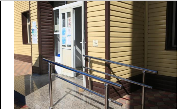
Ramp in Building 4
