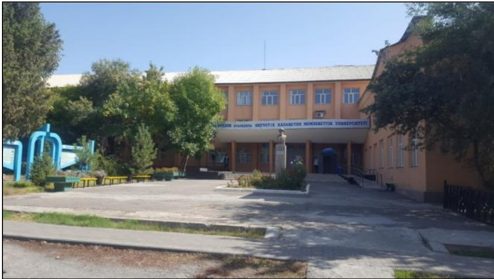
Campus 5, Central entrance to building 9 (M.Auezov SK University, Kazakhstan)
