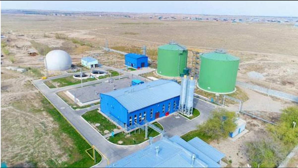
The final stage of water purification
